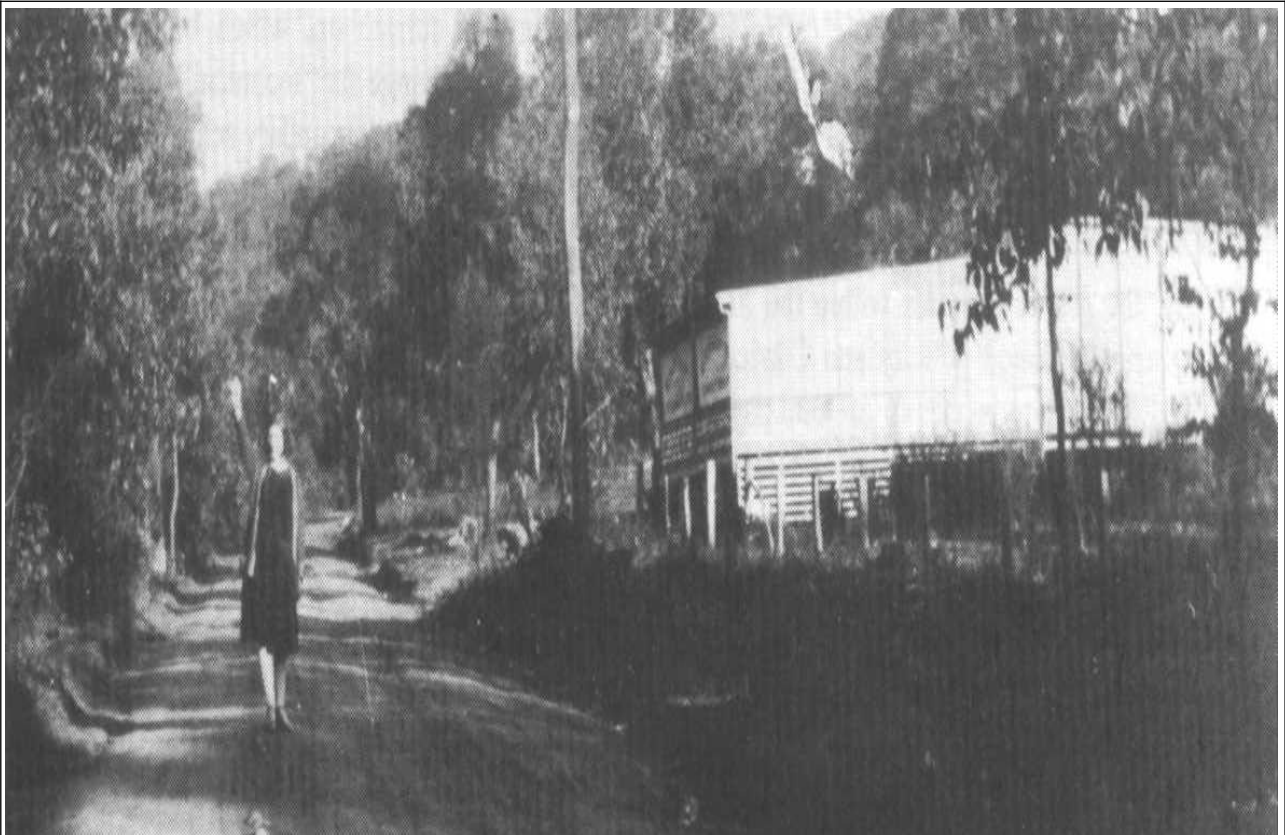
Rear of Canes Store. Circa 1933. The attached "Glideaway Hall" is on the right. Both were demolished in the 1970's. Eileen Turner standing on the 1 in 20 Road (later Mountain Highway).
