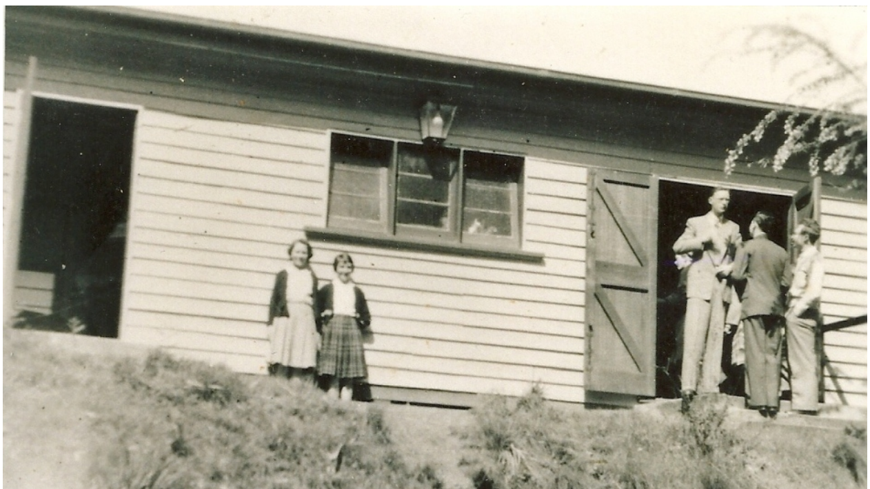
The Basin Presbyterian Church on the corner of Church Street and Forest Road c1954. Helen Johnson, Glenys Greenwell, Dick Heyliguis, Alan Henley, Linton Hersfield. In 1964, this building was sold to The Basin Scouts and in 1972 it was destroyed by fire. Photo courtesy Knox Historical Society
