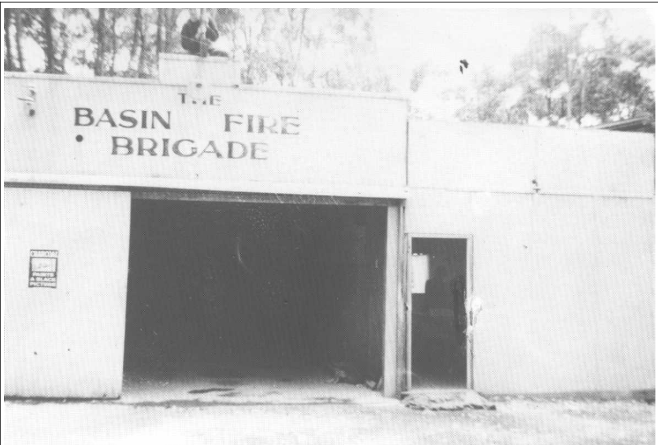
The Basin Rural Fire Brigade second building built in 1953 by voluntary labour on Forest Road opposite the Triangle. Doug Greenwell fixing flagpole on top of building. Photo courtesy Elsie Greenwell.
