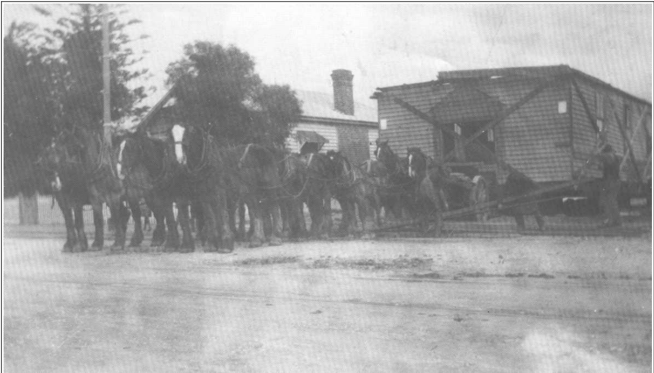
A grain store was purchased for use as a barn by R. B. Smith and carted to The Basin by a team of horses. Circa 1926. Photo shows the building ready for hauling by a team of nine horses.
