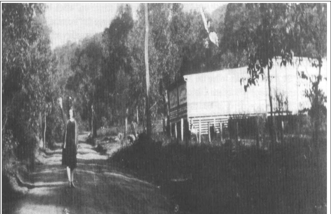
Rear of Cain’s Store. Circa 1933. The attached “Glideaway Hall” is on the right. Both were demolished in the 1970’s. Eileen Turner standing on Mountain Highway. Photo courtesy Eileen Turner.
