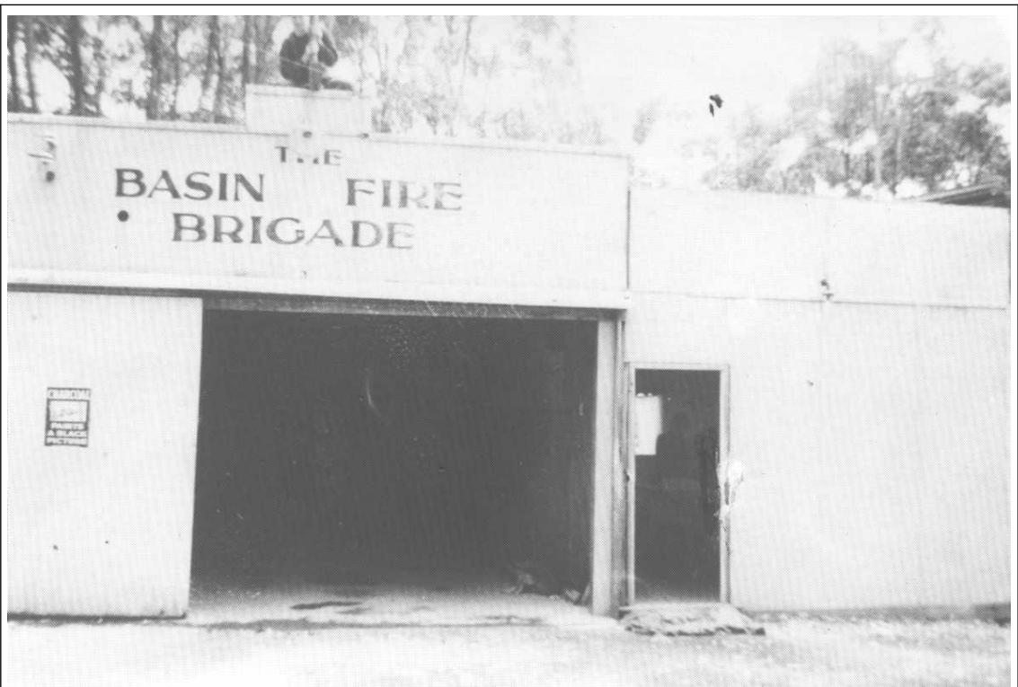
The Basin Rural Fire Brigade second building built in 1953 by voluntary labour on Forest Road opposite the Triangle. Doug Greenwell fixing flagpole on top of building. Photo courtesy Elsie Greenwell.
