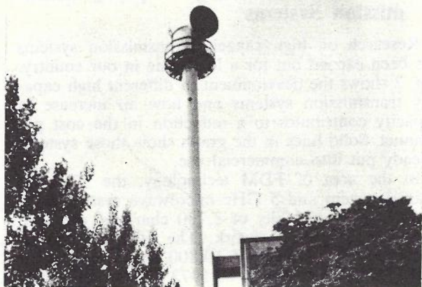
Fig. 3—Repeater station of a quasi-millimeter wave radio system
