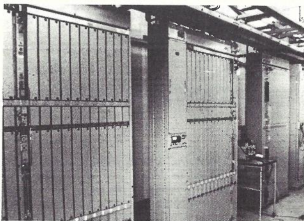
Fig. 4—Repeater station of a guided millimeter wave system
