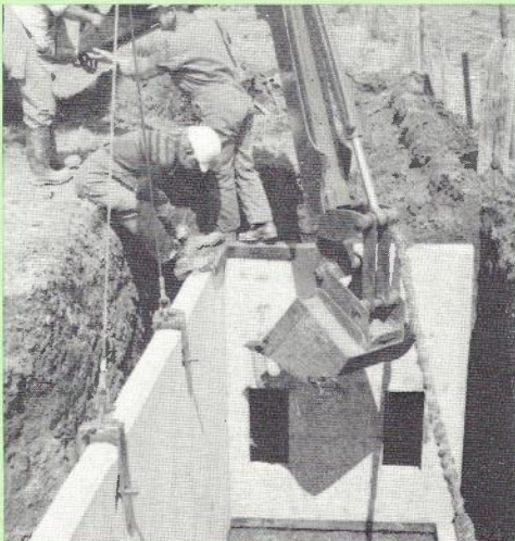
Installation of PF20 manhole
