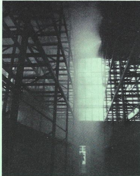
Discharge tests of the automatic sprinkler system especially designed for the high rise warehouse racking – Supply Branch, Springvale.
