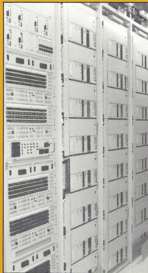
NEC Type Rack (Left) Type 72 Racks with PCMME Equip't.
