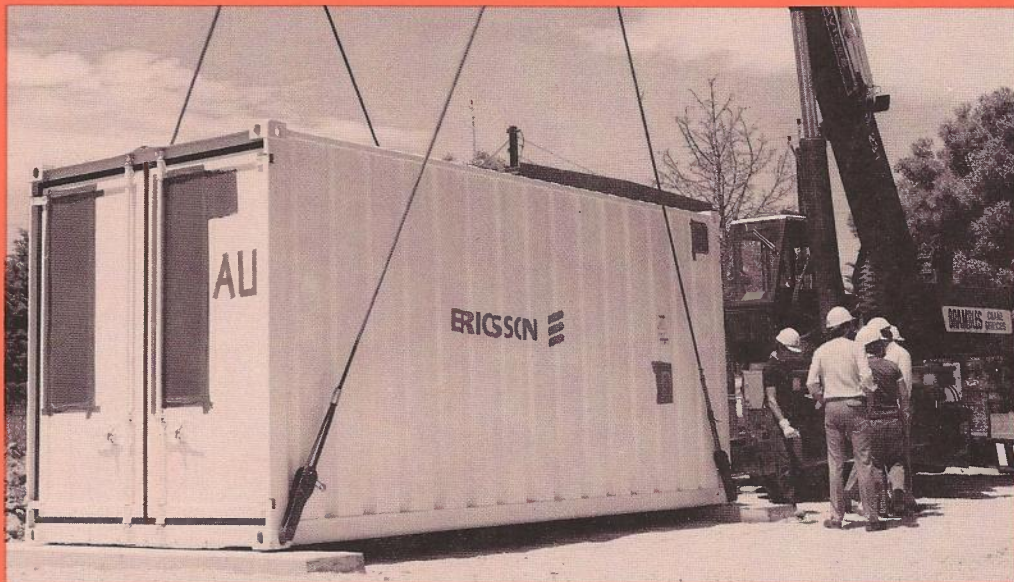
L. M. ERICSSON CONTAINER BEING SITED AT ONE TREE HILL S.A.
