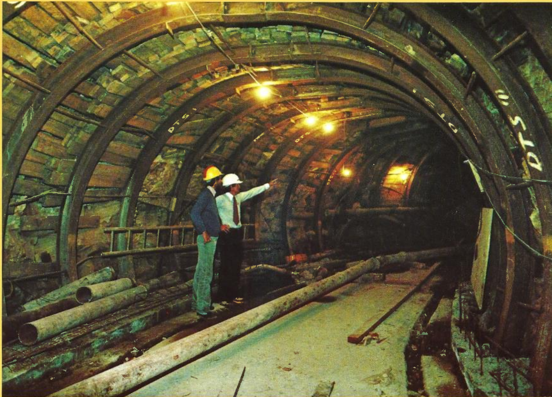
Steel supports to double width of tunnel, Exhibition St.
