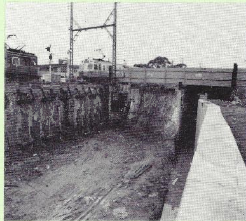
Station St. end of excavation.
