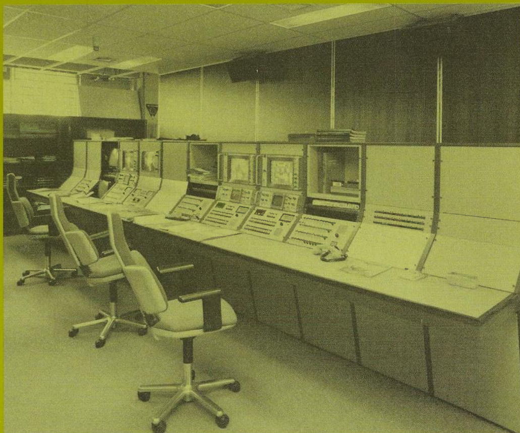
Control Suite at Surrey Hills Radio Terminal
