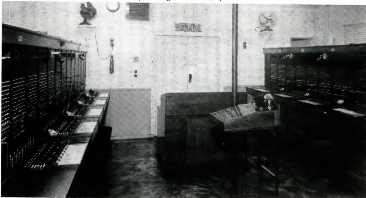
Fig. 3.5 — Queanbeyan Exchange 1954 CBM Local and Sleeve Control Trunk Positions.
