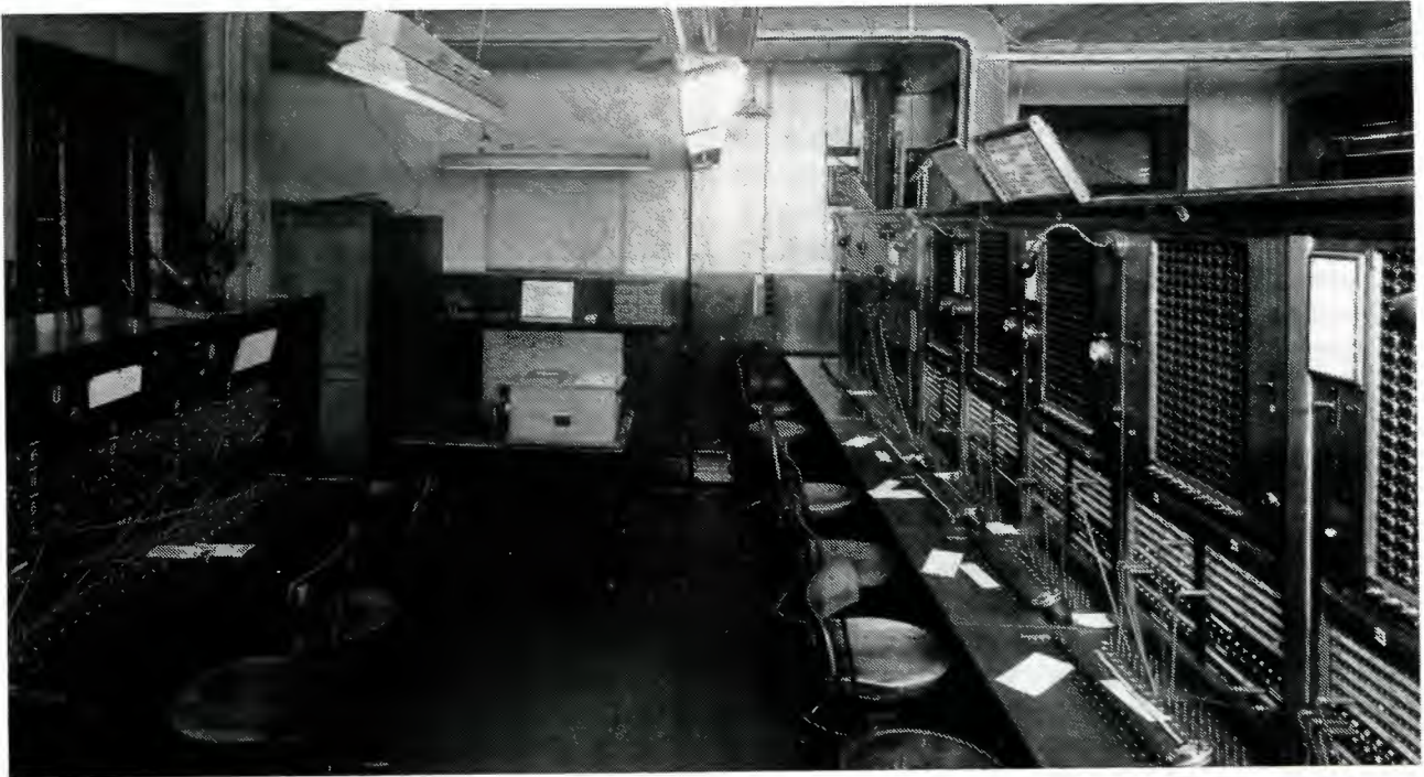
Fig. 2.4 — Hamilton Exchange, NSW non multiple magneto A positions series multiple B positions
