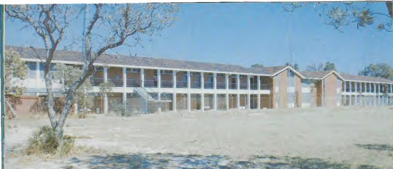
Above: Technical Training Centre, Manning, Western Australia.
