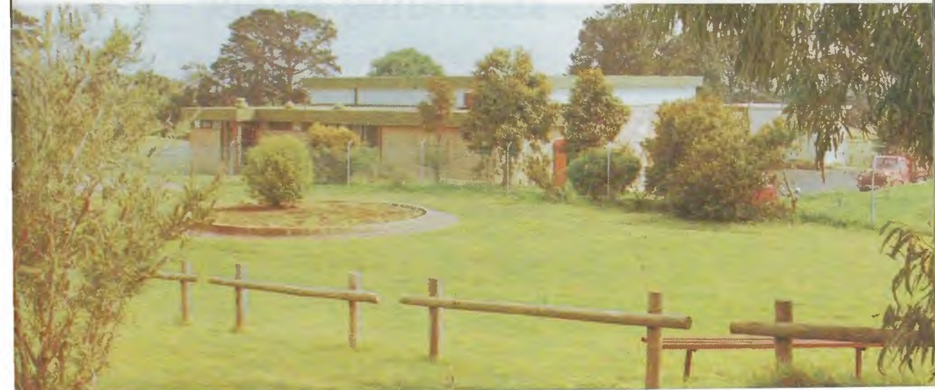
Below: Terminal telephone exchange, Karingal (Vic).
