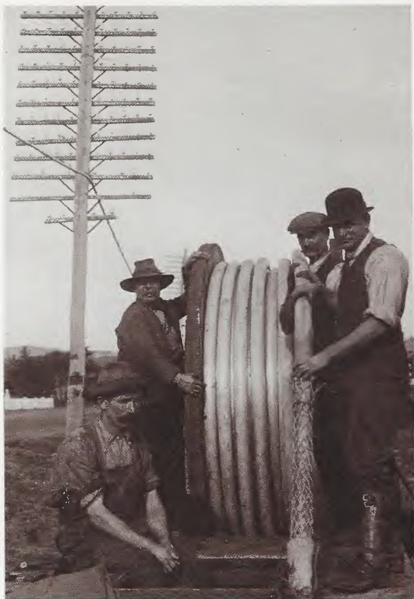
Cable hauling – Perth to Fremantle, Western Australia, 1916.
