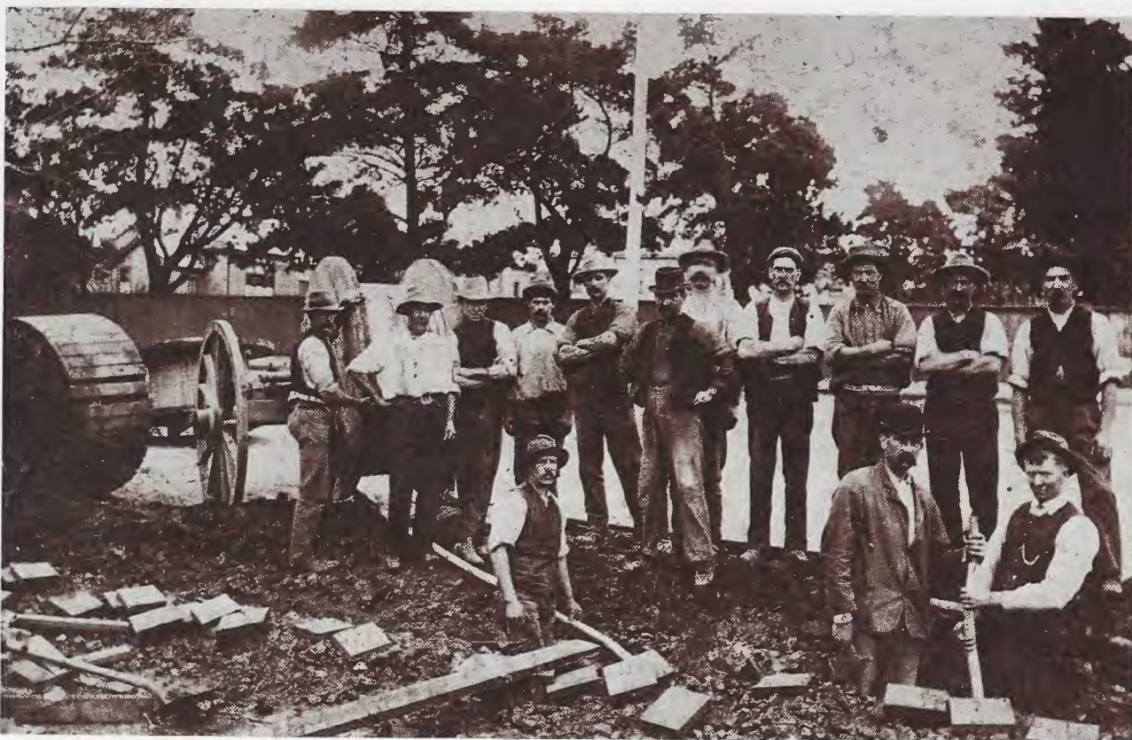
Laying the first underground cable in Geelong, 1912.
