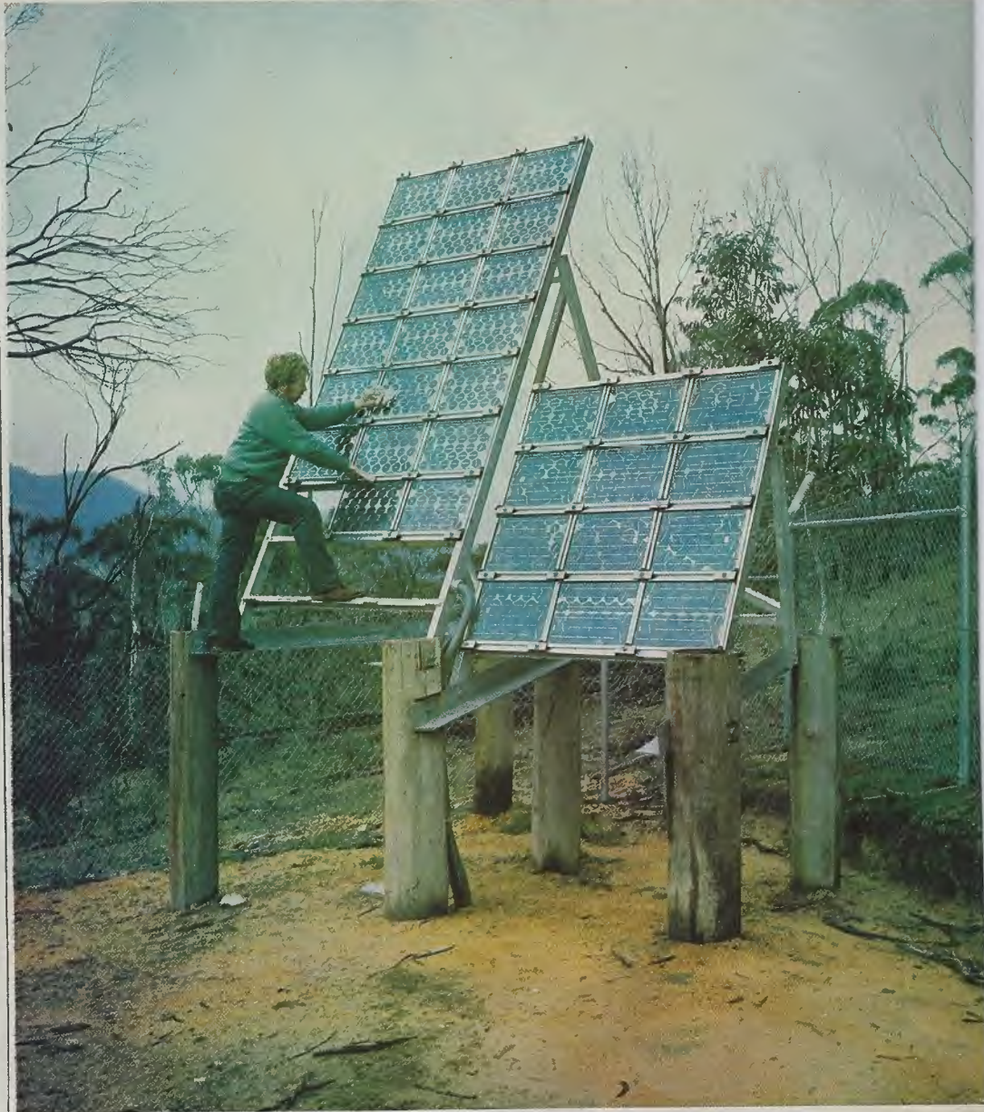
Cleaning the cells on a solar-powered system.
