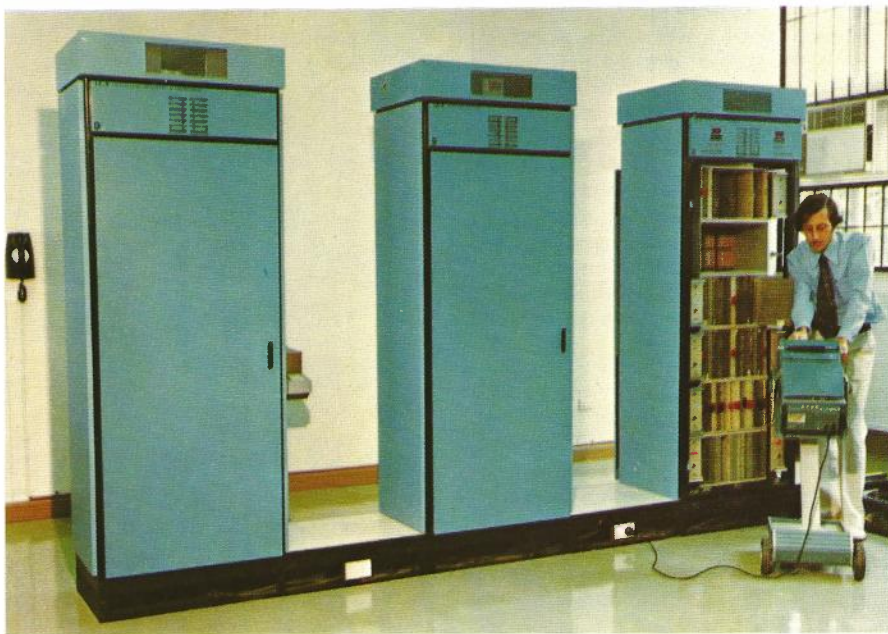
The model 1ST exchange at St. Kilda showing equipment cabinets
