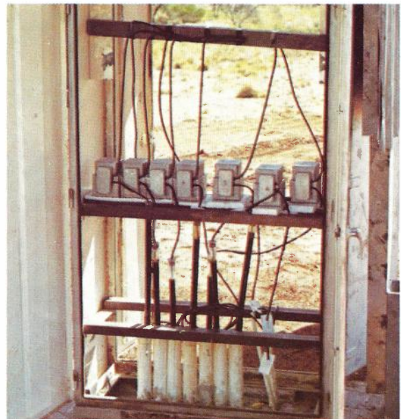
Lightning voltage counters on Port Hedland to Mount Newman coaxial cable
