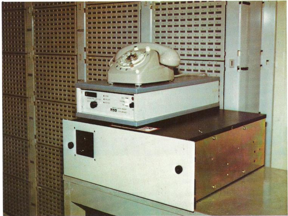
The microprocessor metering system installed in a suburban telephone exchange
