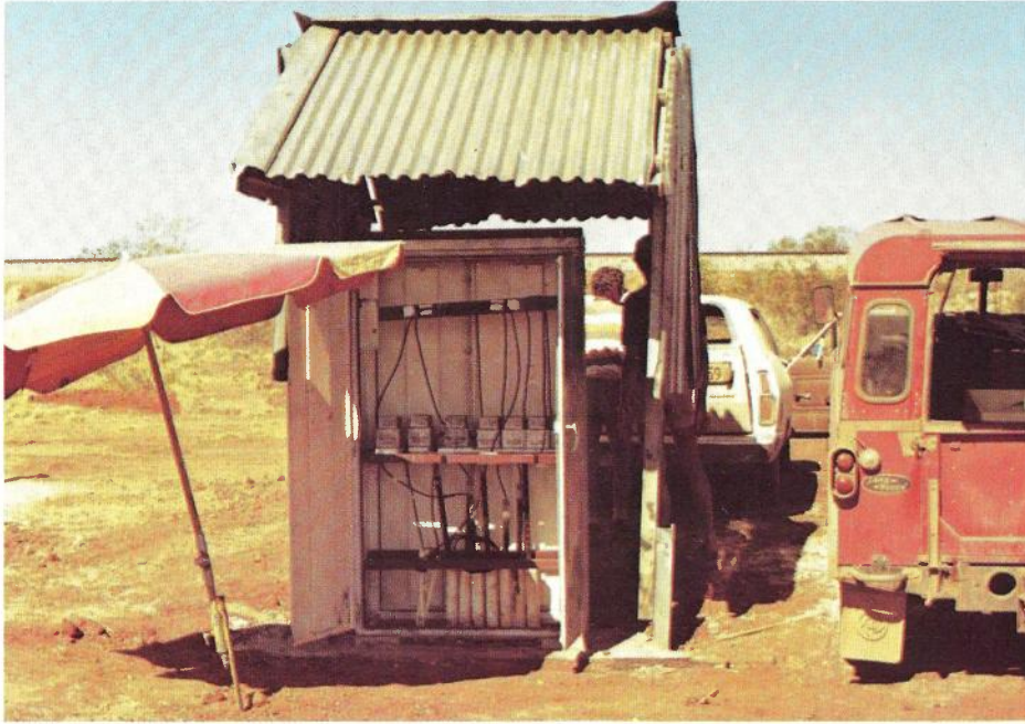
Lightning voltage counters on Port Hedland to Mount Newman coaxial cable
