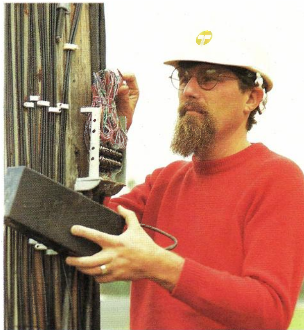
A Laboratories' scientist examines insulation on cable conductors terminated in an above-ground joining enclosure
