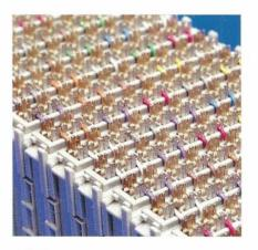
**Above** Part of an MDF module, showing insulation displacement terminals
