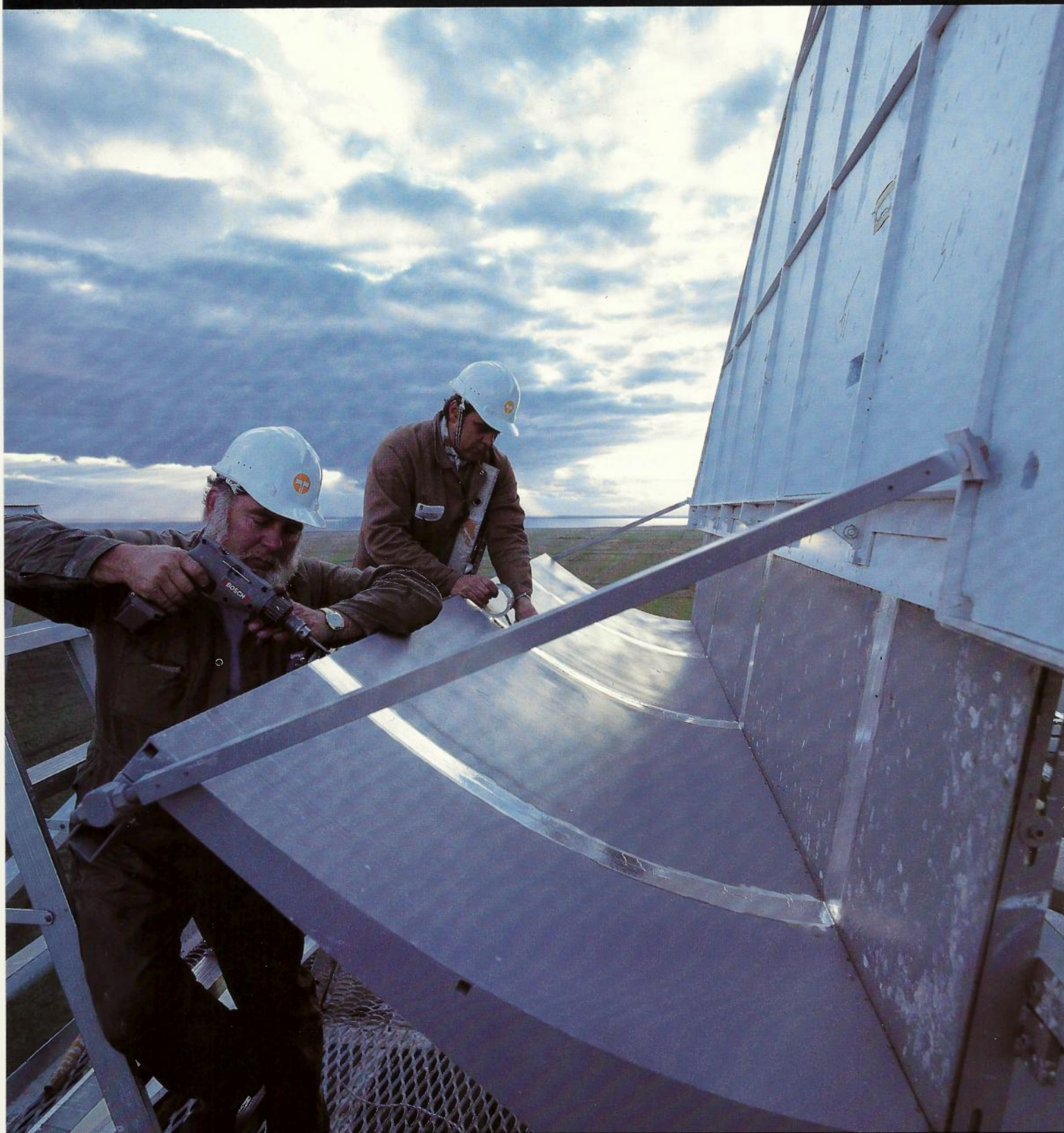
Researchers, Barry Gilbert and Doug Farr adjusting and assembling a High Resolution Antenna at Telecom's Caldermeade Antenna Test Range.
