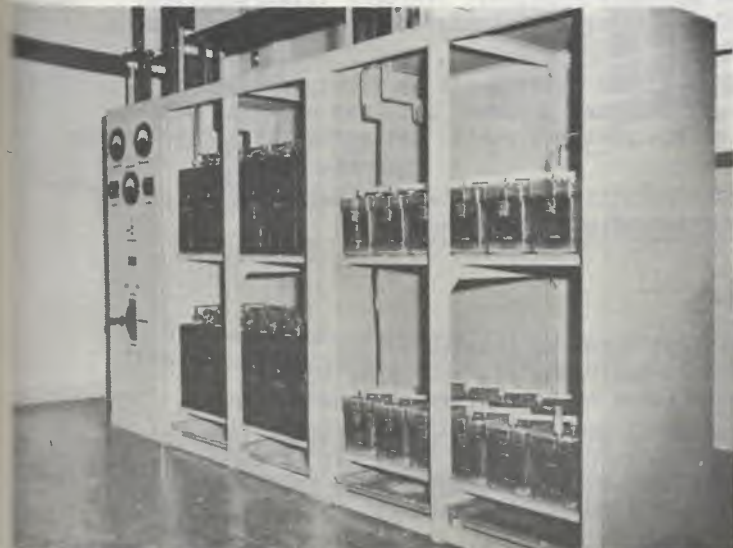
FIG. 18. 6 VOLT ACCUMULATOR ENCLOSED TYPE, HARD RUBBER CONTAINER.
