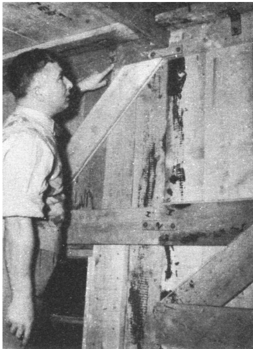
FIG. 7. PORTABLE BUILDING - TEMPORARY STORAGE UNIT. (Showing Assembly Method)
