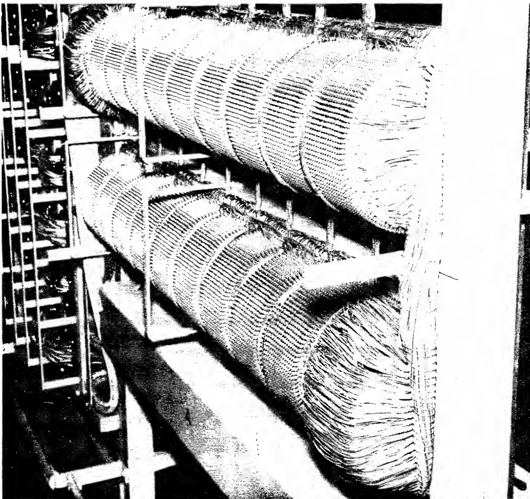
FIG. 2. BANK MULTIPLE CABLING.
