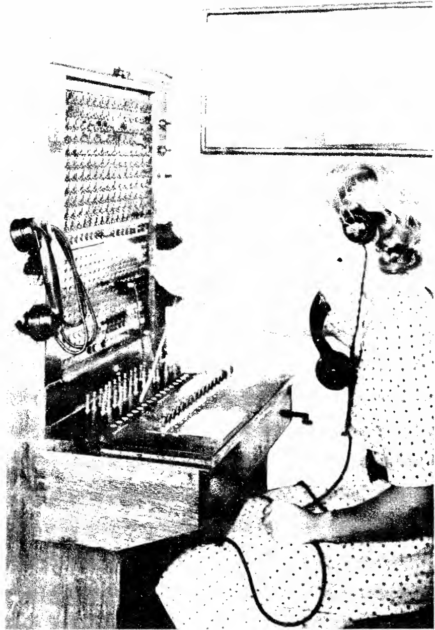
MAGNETO FLOOR PATTERN SWITCHBOARD.
