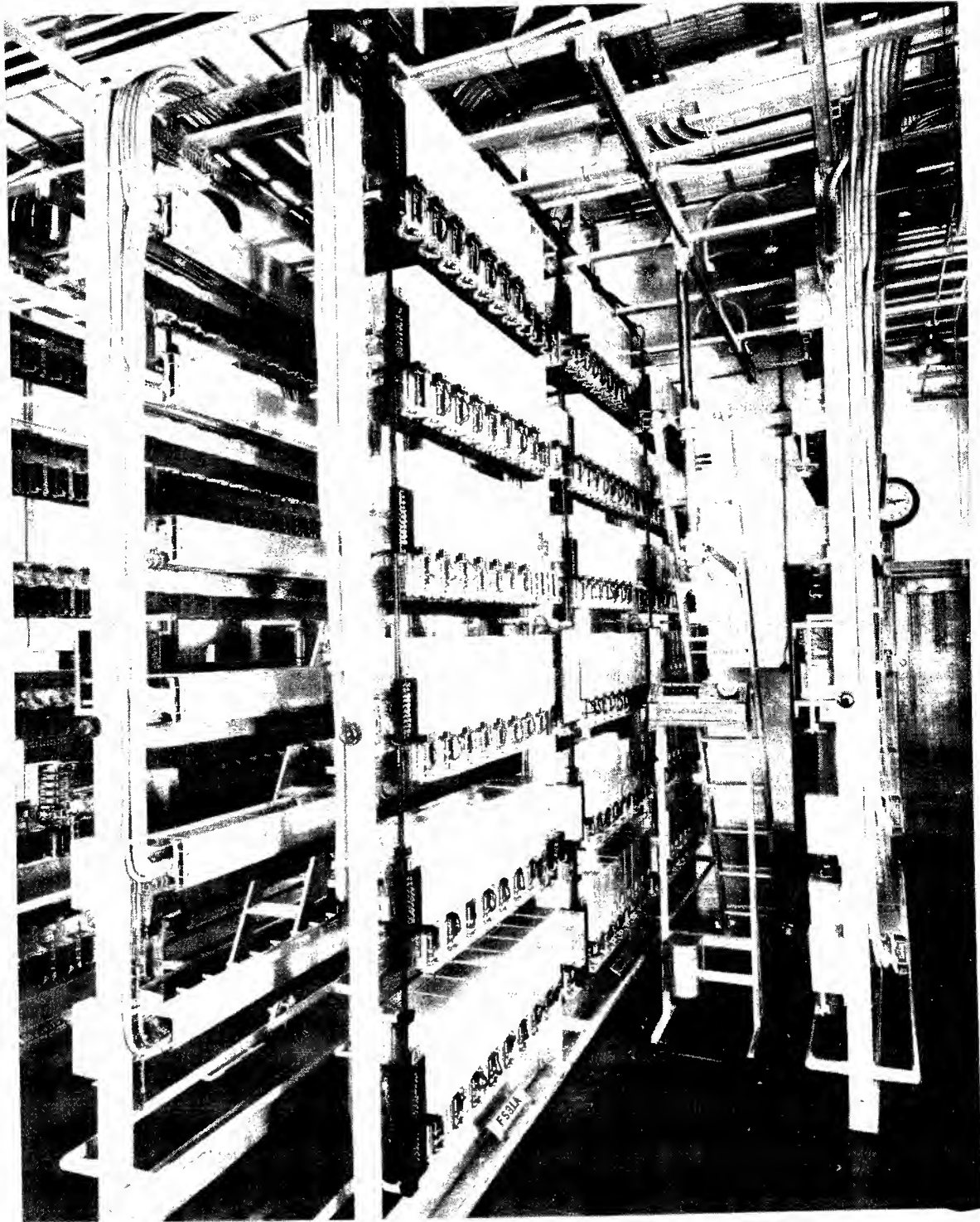
SUITES OF FINAL SELECTORS SHOWING WIRING AND APPARATUS AISLES.
