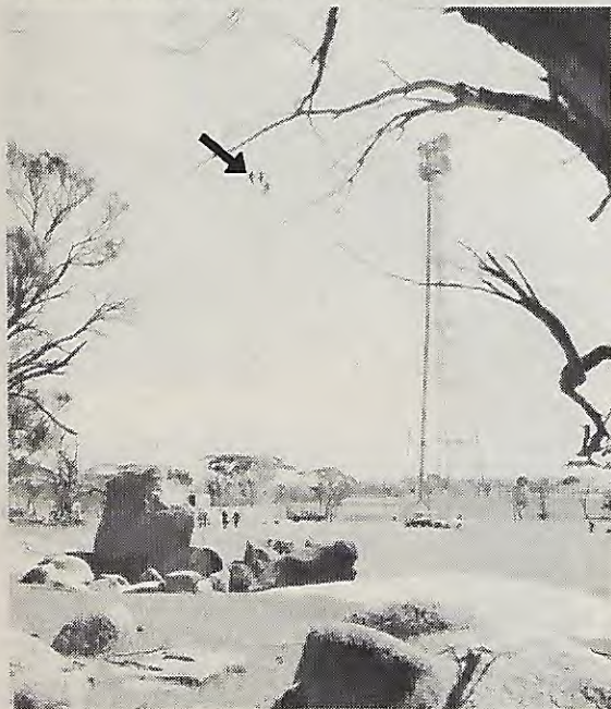
WA Telecom engineers don't intend to be caught unprepared by future cyclones. Here at Bulgin Rock near Meckering they practice erection of zip-up microwave masts to replace damaged towers. Arrow indicates men on Jury mast.
