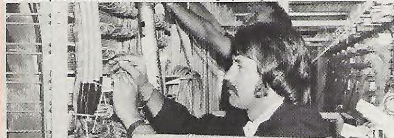
Technician Paul Hill wires a switch bay in the new Exchange building.
