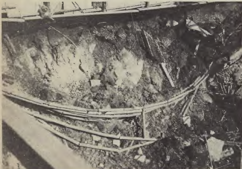
Dangerously sagging cables pictured just after the wall collapse. The main Melb.-Syd. co-ax is seen second from the bottom.
