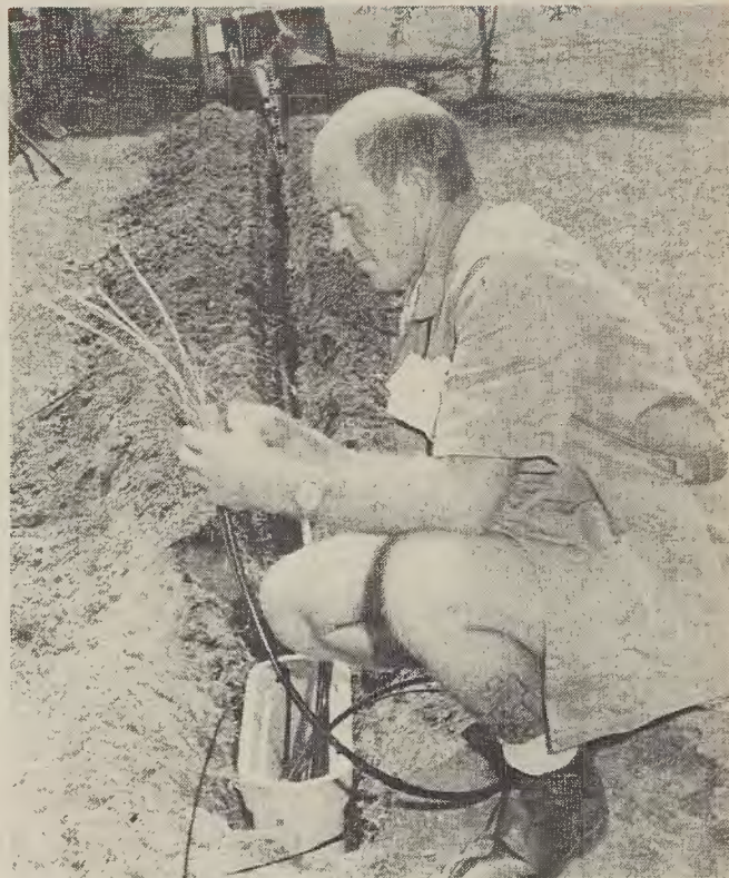
Highly visible in the connection process: cable jointer Brian Fitzjohn connects a wire pair from Mrs Rosenbaum's home to a new 10-air cable just installed in the street outside her home. Ditcher operator, Cyril McPhail covers the new cable. Below: Part of the work which has sprung from forward planning — Glen Allard connects a new 400-pair main cable (newly installed on the railway bridge across the Macleay) to a main distribution cabinet. Once he has completed his work the cabinet will serve 300 new connections in South Kempsey.
