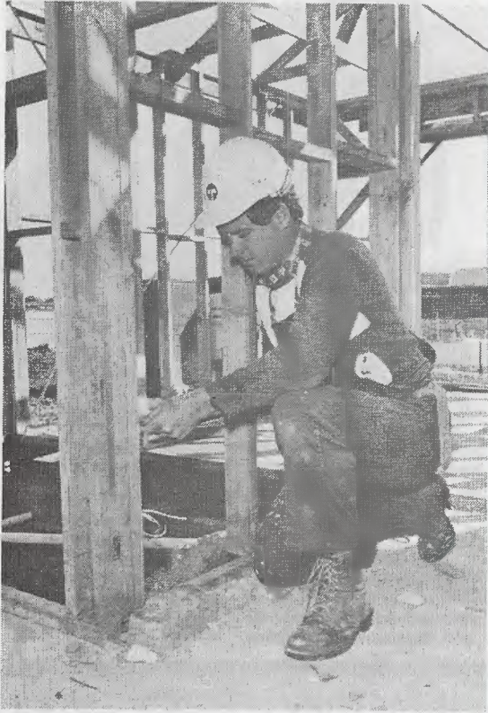
Terry Craig, Serviceman-in-training, fits a clipsal bracket for a telephone point in the HIA (Vic) 1981 Apprentice House of the Year, Carrum Downs, Victoria.
