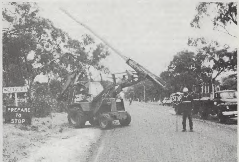
The poles are removed by specially equipped tractors and loaded into trucks.
