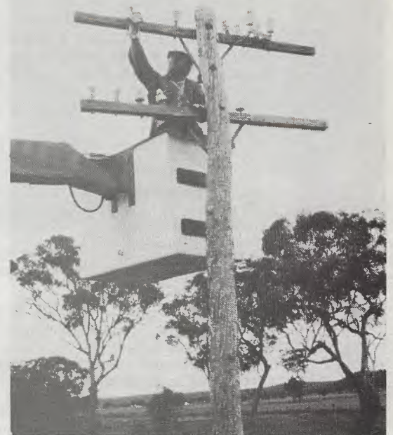
The ABBEY crew undo the braces and combiners and cut the stay wires.
