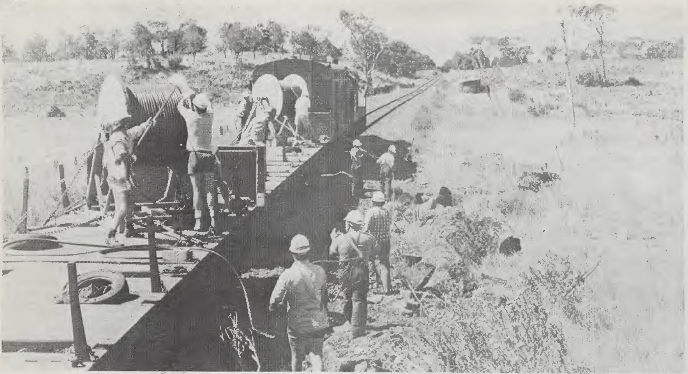
● Colac External Plant staff dispense aerial cable in the Stoney Rises area.
