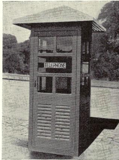
Fig. 6.—Tropical Type Cabinet Installed in Queensland.
