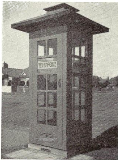
Fig. 1.—Former A.P.O. Standard Cabinet, mounted on "cast in situ" Concrete Base.
