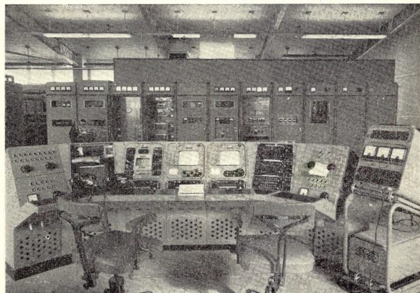
Fig. 11.—Transmitter Control Desk and 18 kW Transmitter.
