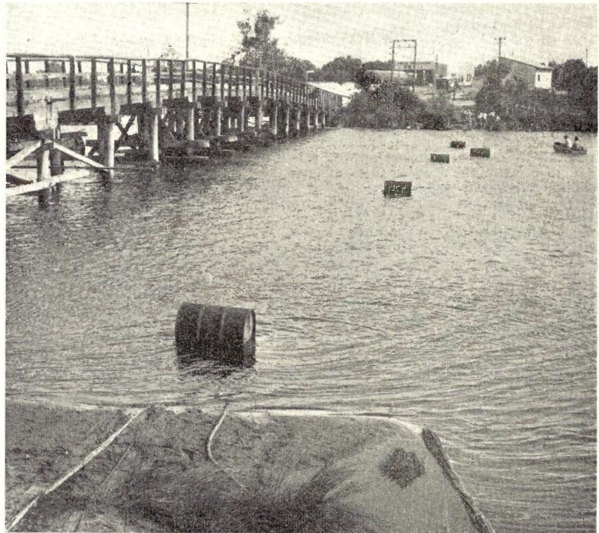
Fig. 2.—View from eastern bank, showing old bridge and cable buoyed prior to plowing in.
