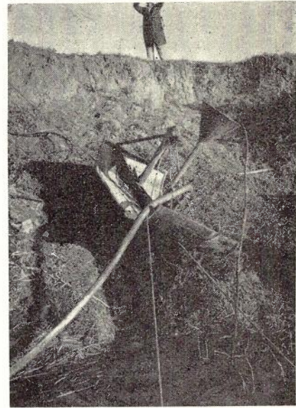
Fig. 4.—Skid Plough Entering River.
