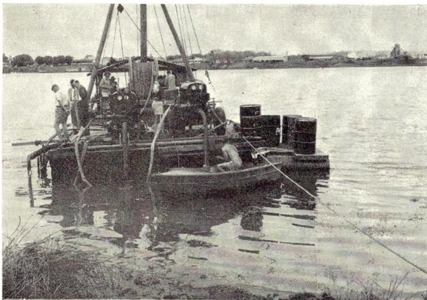
Fig. 8.—Preparing to lay Cable at Grafton.
