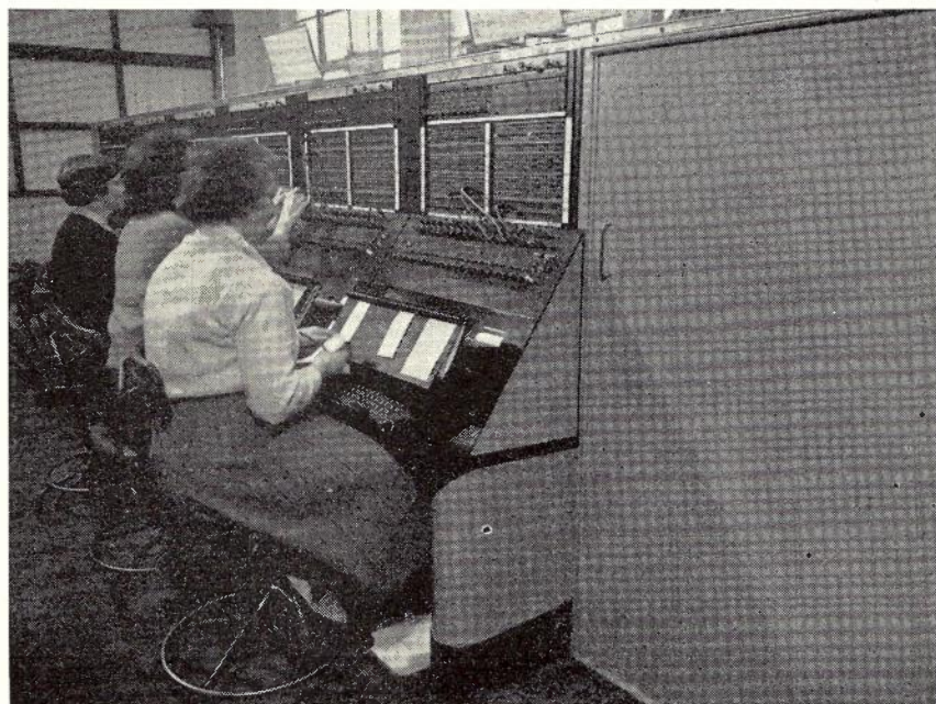
Fig. 5.—Multiple Switchboard Positions.
