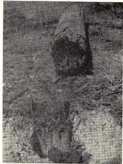
Fig. 11.—Untreated Test Pole Completely Destroyed by Decay and Termite Attack.
