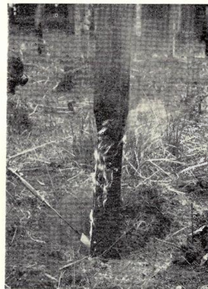
Fig. 4.—Oxyacetylene Charring Process, Charring with Special "T" Jet.
