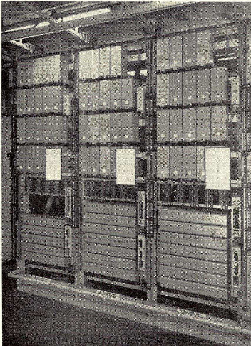
Fig. 12.—Switchboard Rack Equipment.
