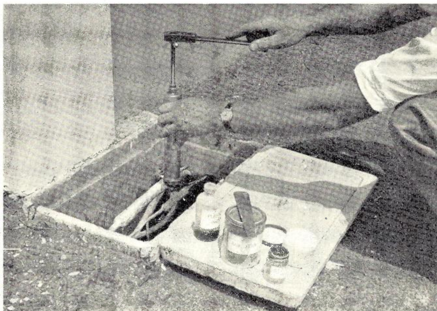
Fig. 4.—Illustrates materials required and method of injection into a "wiped-on" sleeve.
