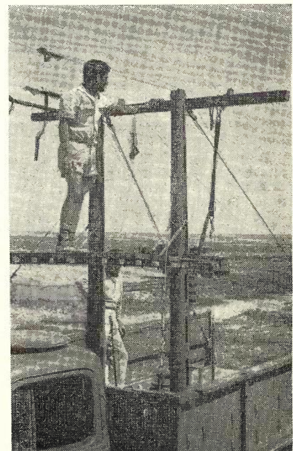
Fig. 9.—Wire Tensioning Truck.
