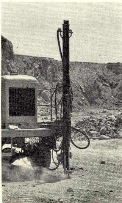
Fig. 8.—Drilling Holes in Rock for Stays.
