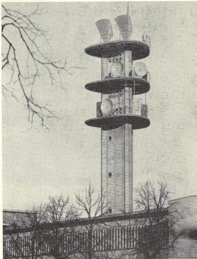
Communication tower of a large station
