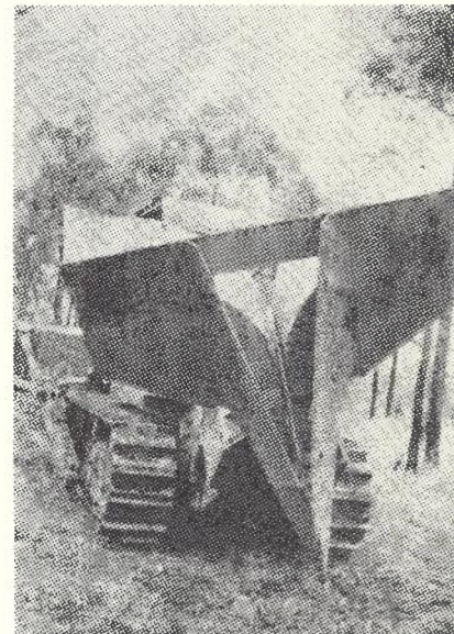
Fig. 9.—Trenching Plough Attached to Back of Tractor.
