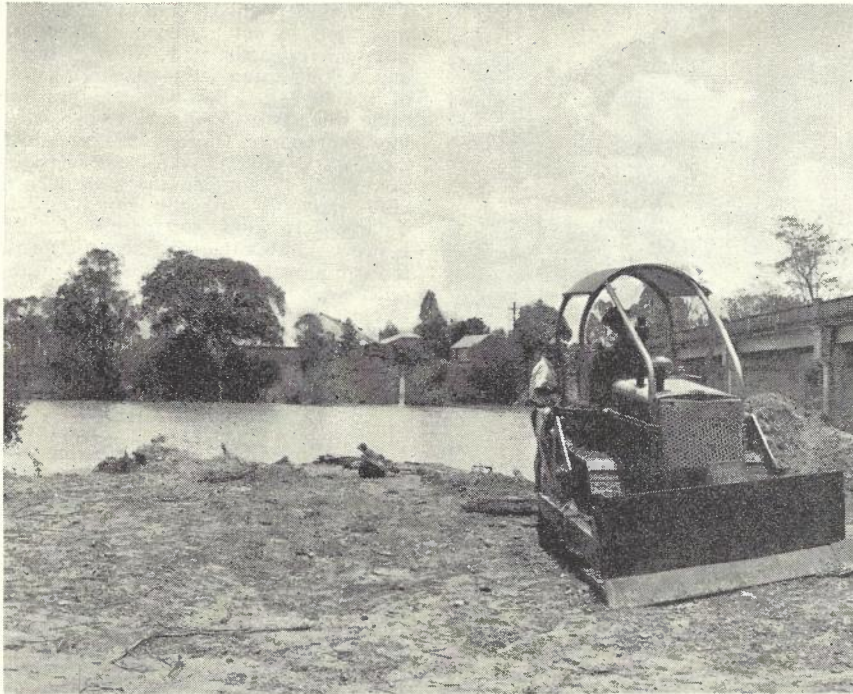
Fig. 2.—Drag Line Excavator and Tractor at the Coomera River.
