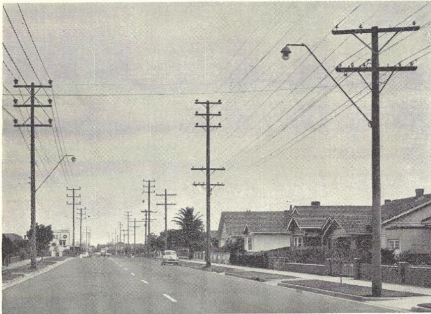
Fig. 2.—High Voltage Lines Flanking Both Sides of Warrigul Road, Melbourne. Such lines introduce the hazard of low frequency induction into the underground telephone cables under earth fault conditions.
