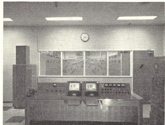
(c) Interior of ABHN-5, Control position looking through to transmitter hall.
