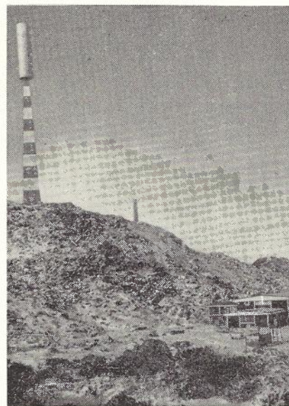
(b) View of erected structure. Fig. 17.—Aerial Radome at Mt. Barrow, Tas.
