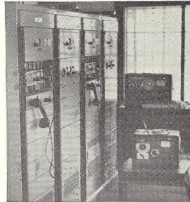
V.H.F. Radio Racks at Kerewan repeater Station, The Gambia.
