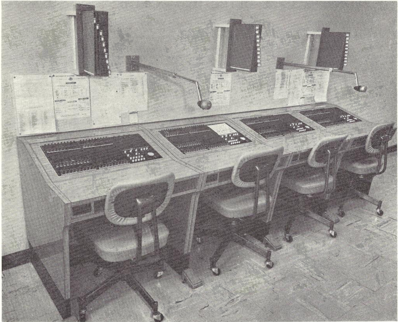
Fig. 16 — Operators' Consoles and Public Address System Microphones
