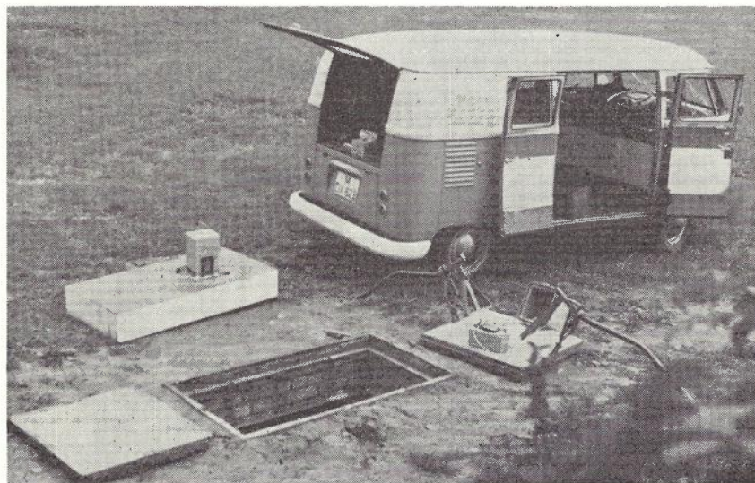
Fig. 2 — Cable Manhole Opened
