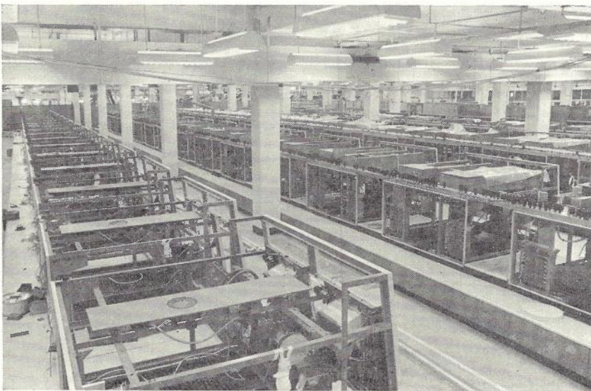
Fig. 3 — General View of Coders Being Installed on 4th Floor.
