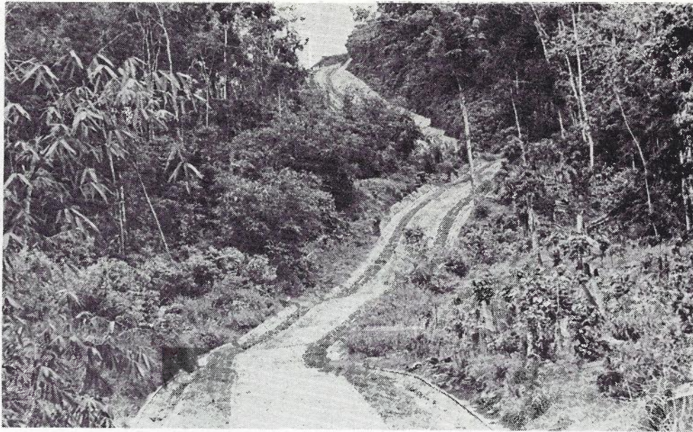
Fig. 5 — TSMS Typical Access Road (during construction stage).
