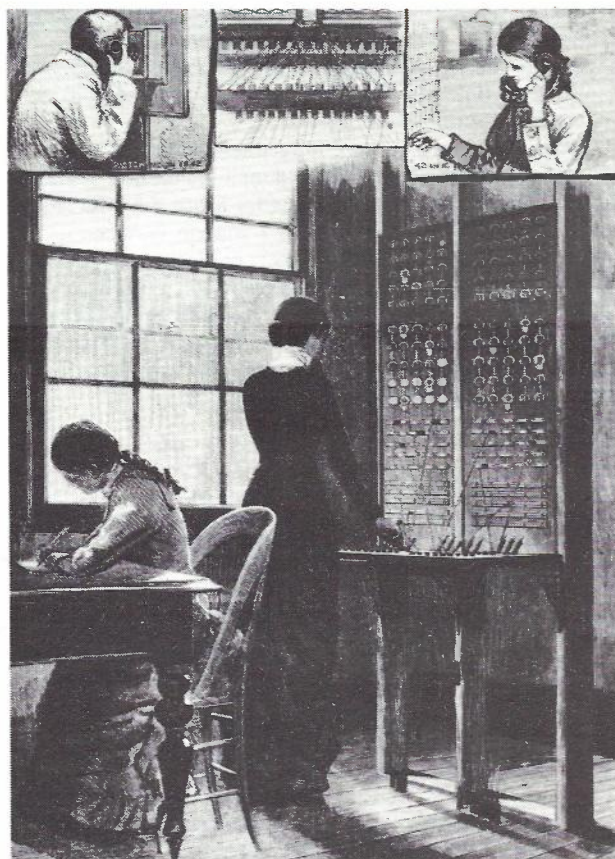
First Telephone Exchange in Melbourne
