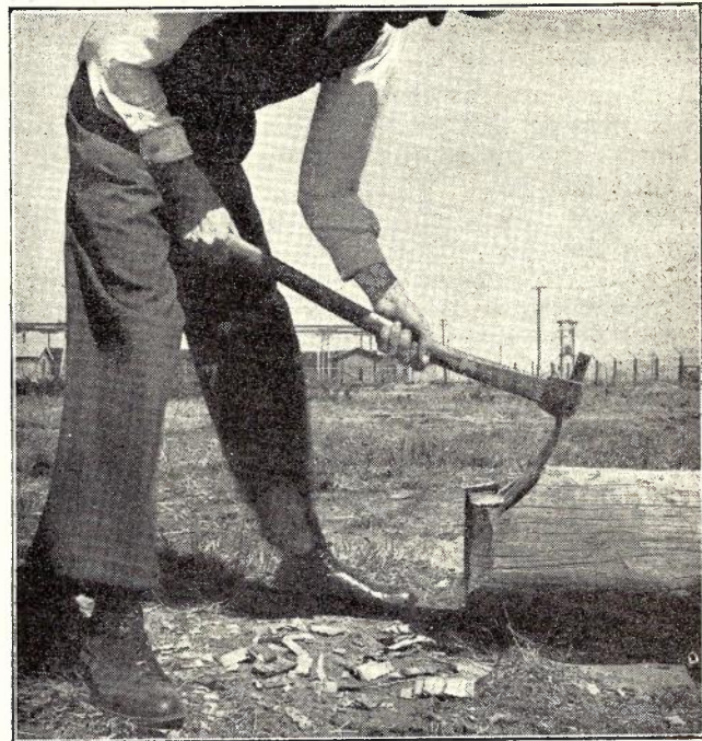
Fig. 10.—Cutting Bevel with Adze.
