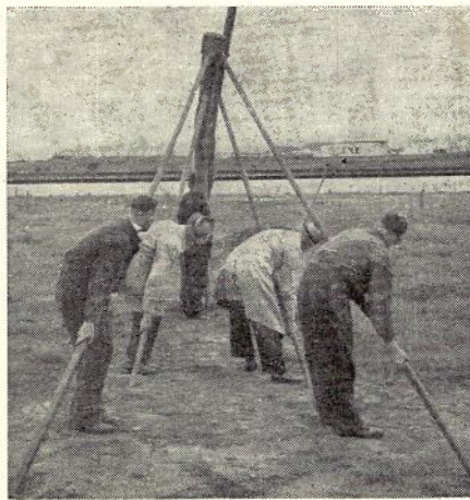
V. Pole Higher: Pikes used for lifting. (Note V spread to keep pole straight.)
