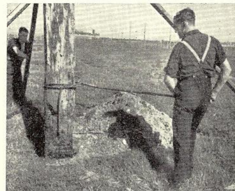
IX. Turning pole with turning rope and sinking bar.
