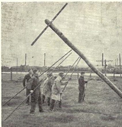
VII. Longer pikes changing to lower position. (Termed "fleeing the pikes.")
