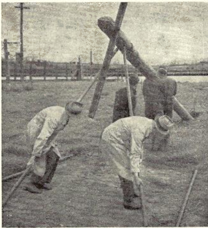
IV. Longer hand pikes take weight and aid lifting.
