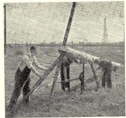
III. Short pikes support pole: Jack does the lifting.
