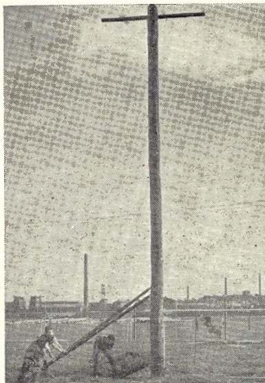
VIII. Final lift: Jack operated in top step of hole.
