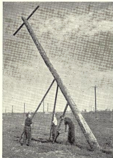
VII. Jack and pikes move down pole in stages.
