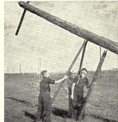
VI. A longer buoy is fitted to jack: Pikes support pole while jack is shifted.
