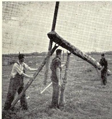
IV. A buoy is fitted in loops on jack to increase effective length.
