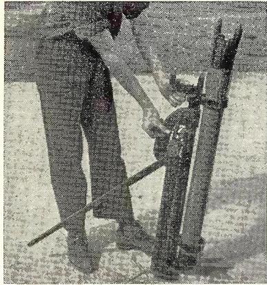
I. Close-up of Pole Lifting Jack.
