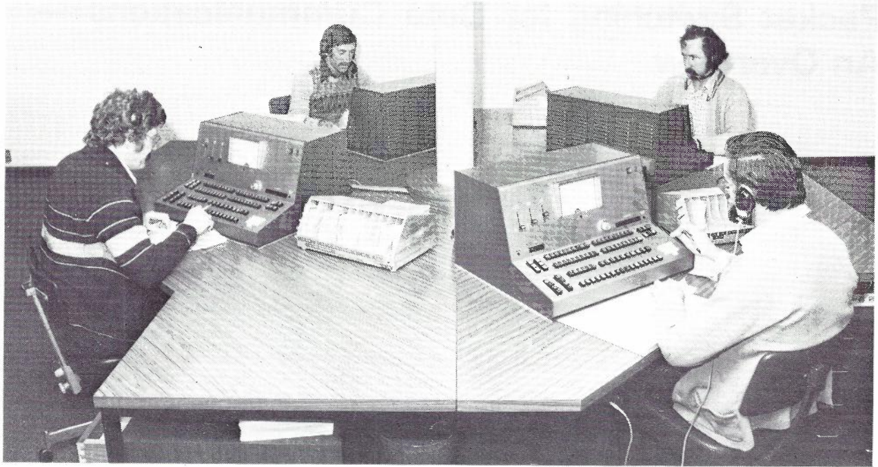
Fig. 5 — Consoles in use at Fault Despatch Centre.
