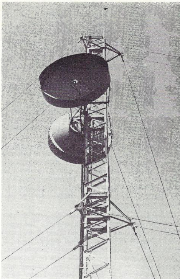
Fig. 7 — Guyed Mast Fixing Arrangements
