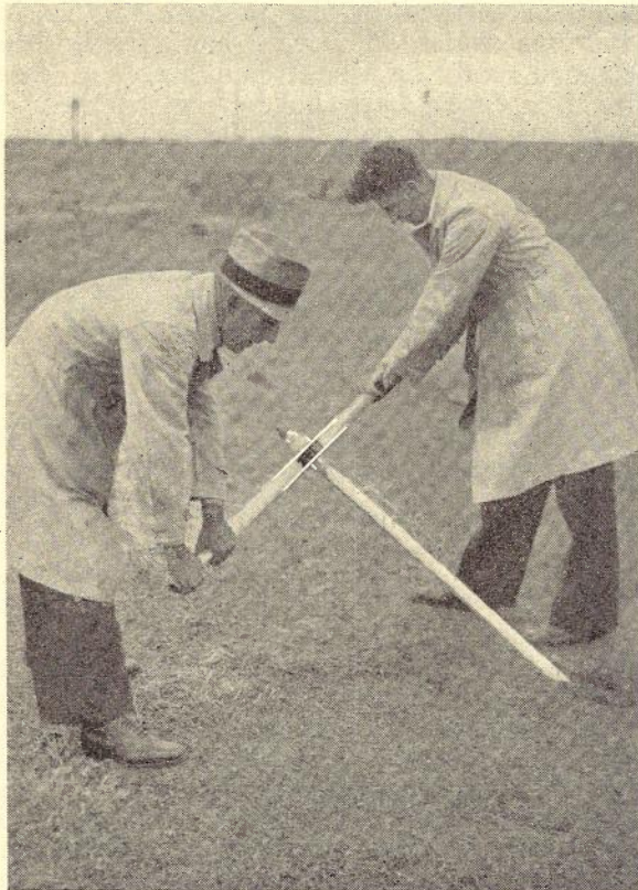
Fig. 99.—Installing Screw Anchor with Ratchet Handle.
