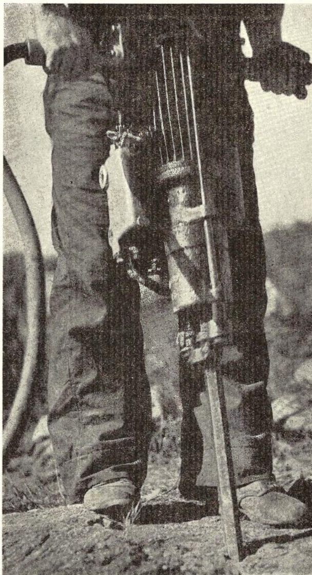
Fig. 33.—Barco Hammer in Use.
