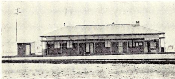
Fig. 8.—Showing the repeater station and P.O. at Rawlinna. This is similar to the other repeater stations between Port Augusta and Kalgoorlie except at Forrest, which is similar to that shown in Fig. 12.
